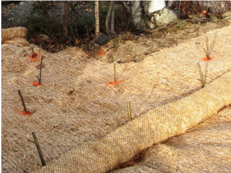
Installation of live stakes
