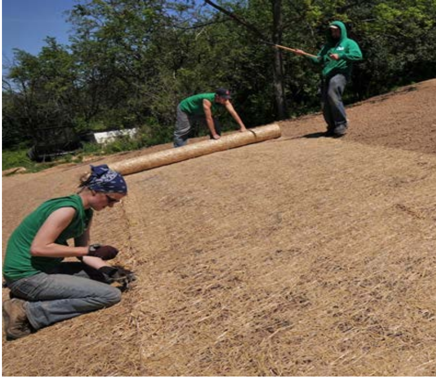
Proper installation for across slope
