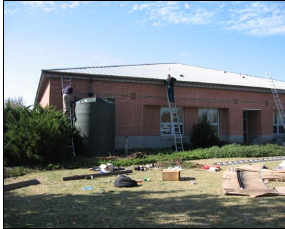
Figure 7.1 3,000-gallon cistern installation in Greenville, N.C.
