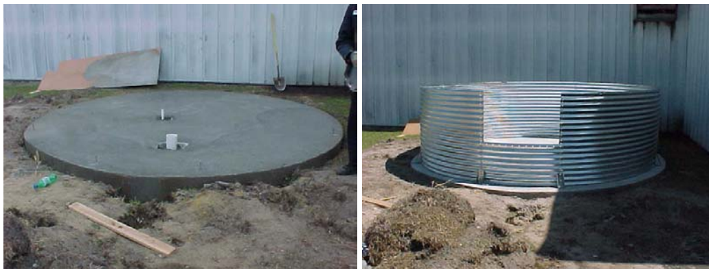
Figure 7.9.a Concrete pad constructed to support (b) a 5000 gallon metal cistern.
