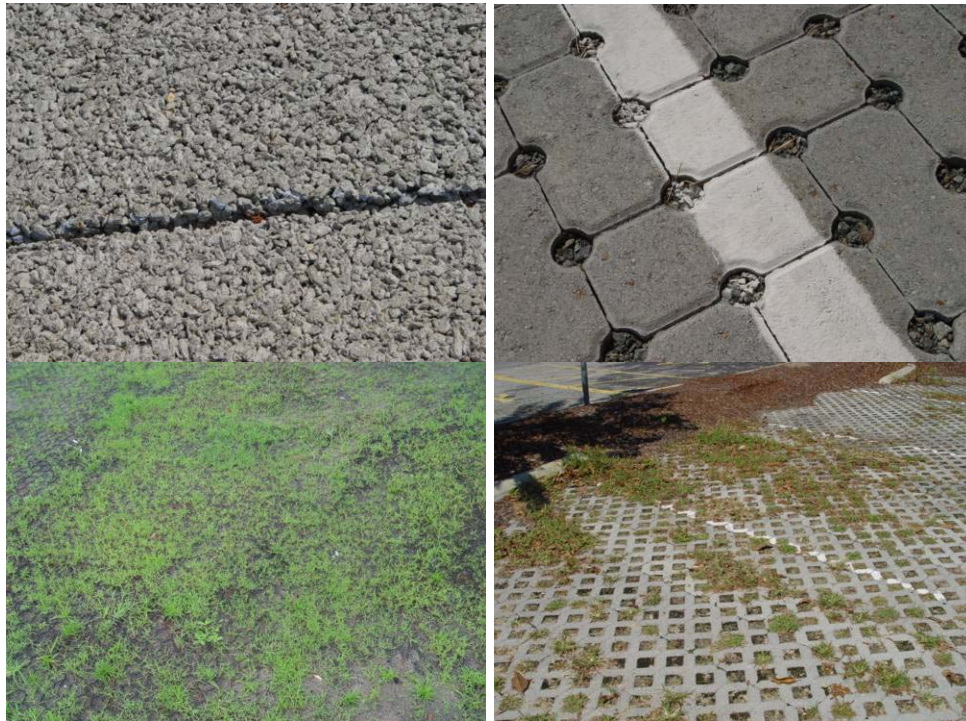
Figure 10.2 Four types of permeable pavements (starting top left corner and moving clockwise): permeable concrete, permeable interlocking concrete pavement, grass pavers, and concrete grid pavers.
