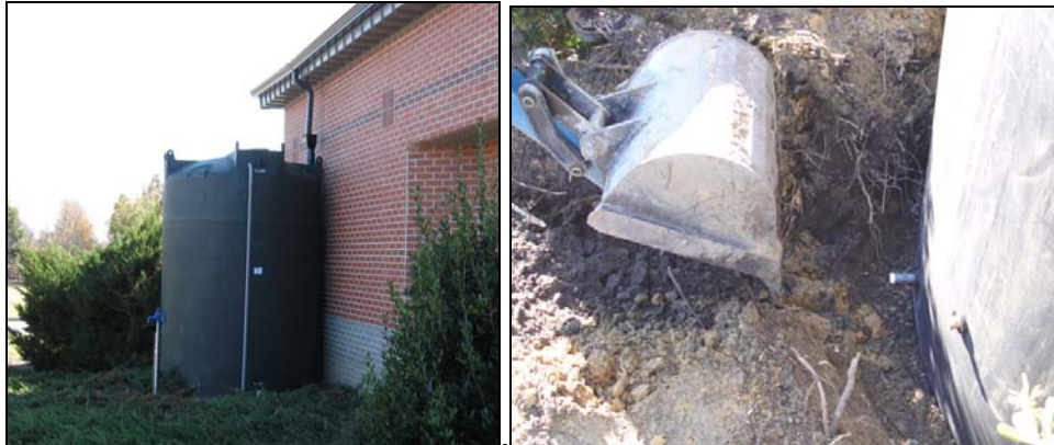
Figure 7.12a Proper cistern placement (b) prepare an area slightly larger than the cistern
