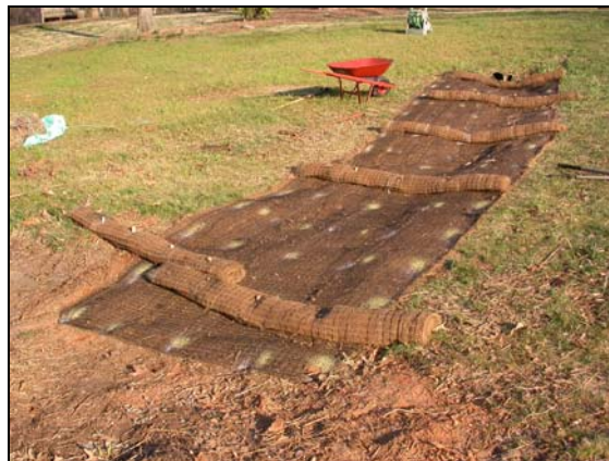
Figure 6.3 Swale leading to BMP with check dams constructed of rolled erosion control matting
