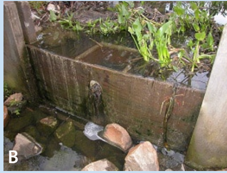
Figure 4. A small orifice allows slow release of captured stormwater (A), but can easily clog due to its size. A clogged orifice can affect plant communities inside the wetland or wet pond (B).
