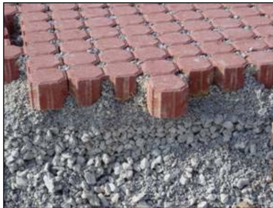
Figure 10.5 Gravel layers under permeable pavers
