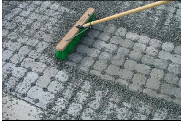
Figure 10.6 Filling permeable paver voids with gravel
