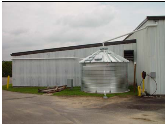
Figure 7.2 5,600-gallon cistern in Kinston, N.C.
