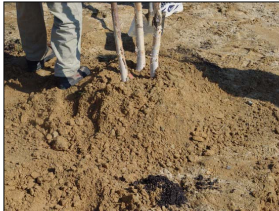
Figure 5.4 Mounding of soil allows certain rain garden plants to survive better in a zoned rain garden.
