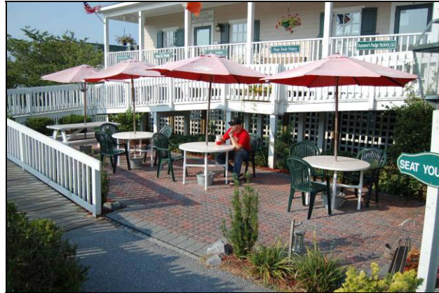
Figure 10.2 Permeable pavement patio outside a café in Swansboro, NC.
