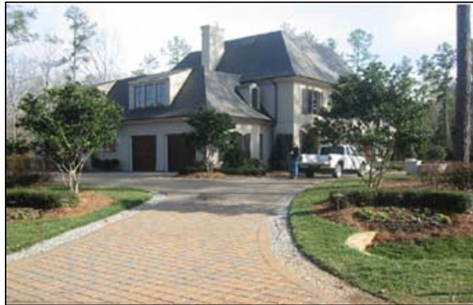
Figure 10.3 Permeable pavement driveway
