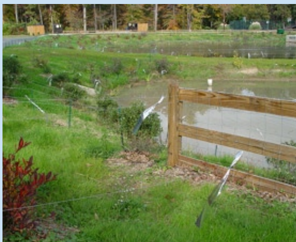
Figure 10. A grid of fishing line adorned with silver tape has been strung across this wet pond to prevent geese from making it their home. The string grid makes water landing more difficult, and geese do not like shiny or flashy objects like wind-blown silver tape.
