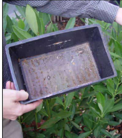
Figure 7.11 Cistern screen close-up
