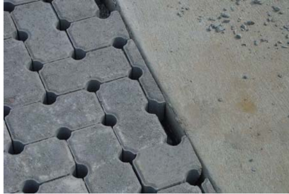
Figure 10.4 Pavers abutting a concrete edge.
