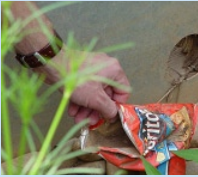
Figure 5. Trash floats to the drawdown hole, where it can clog the small hole, restricting flow. Removing the trash is often very simple, but essential.
