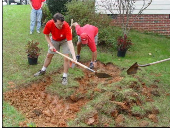
Figure 6.7 Berm Construction at downslope edge of BMP
