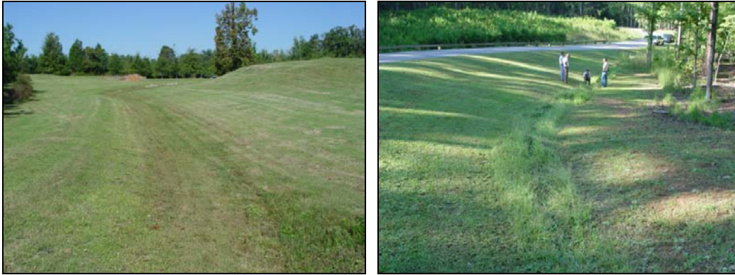
Figures 8.1a and 8.1b show two swales in the Raleigh-Durham area. Both have turf reinforcement mats. The former in Durham (b) is mowed while the latter in Raleigh (a) contains a taller grass stand.
