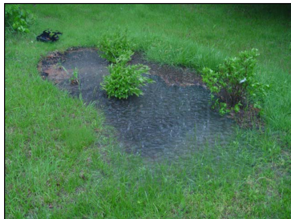
Figure 5.3 First flush events completely fill a rain garden to a ponding depth of 6 inches
