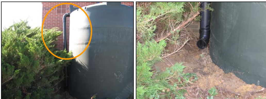
Figures 7.6 and 7.7 Overflow assembly on cistern
