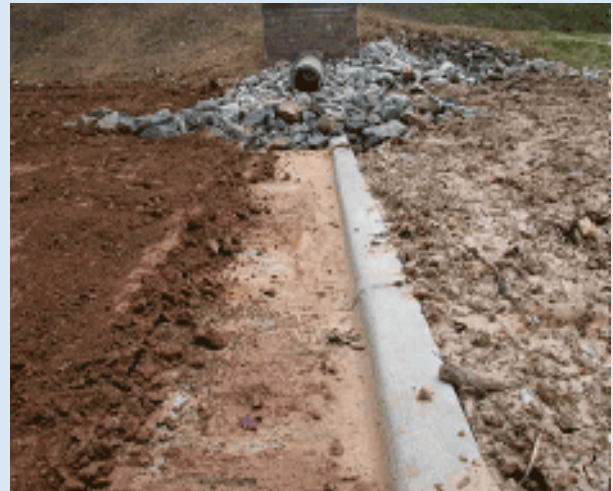
Figure 6. Level spreader just after construction
