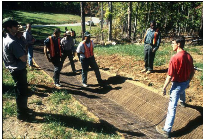
Figure 8.3 Turf reinforcement mats used along a swale at Umstead State Park.
