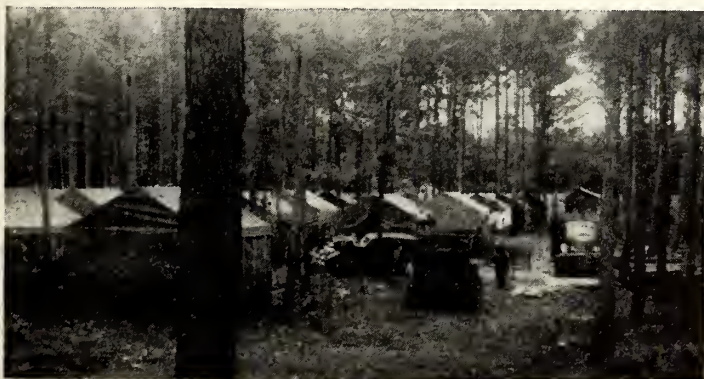
(a) This 1942 temporary farm labor camp was located in Beaufort county near Aurora. It was furnished by the Farm Security Administration and managed by the U. S. Employment Service during the spring harvest season. This was a new venture in this state that proved to be highly approved but was too soon terminated by discontinued federal funds. It accommodated about 600.
