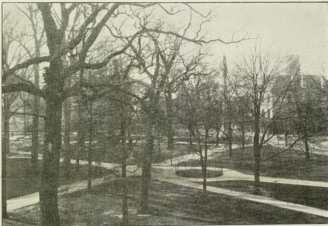
Capitol Square from Department of Agriculture Building. Scene from the Crop Reporting Service office, looking south.
