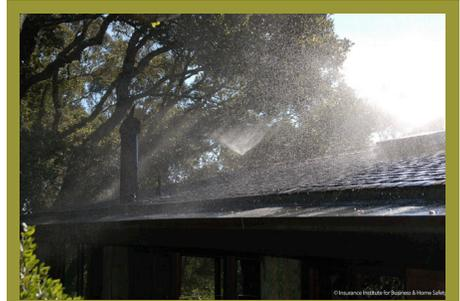
**Photo 1.** Roof mounted sprinkler.
