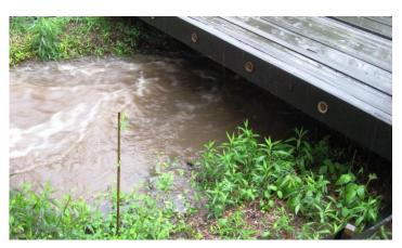
Photo above from April 2012 during a bankfull event at the bridge crossing. The crossing provides ample vertical and lateral clearance for accommodating normal bankfull flow while still allowing NCFS to fully access the State Forest.
