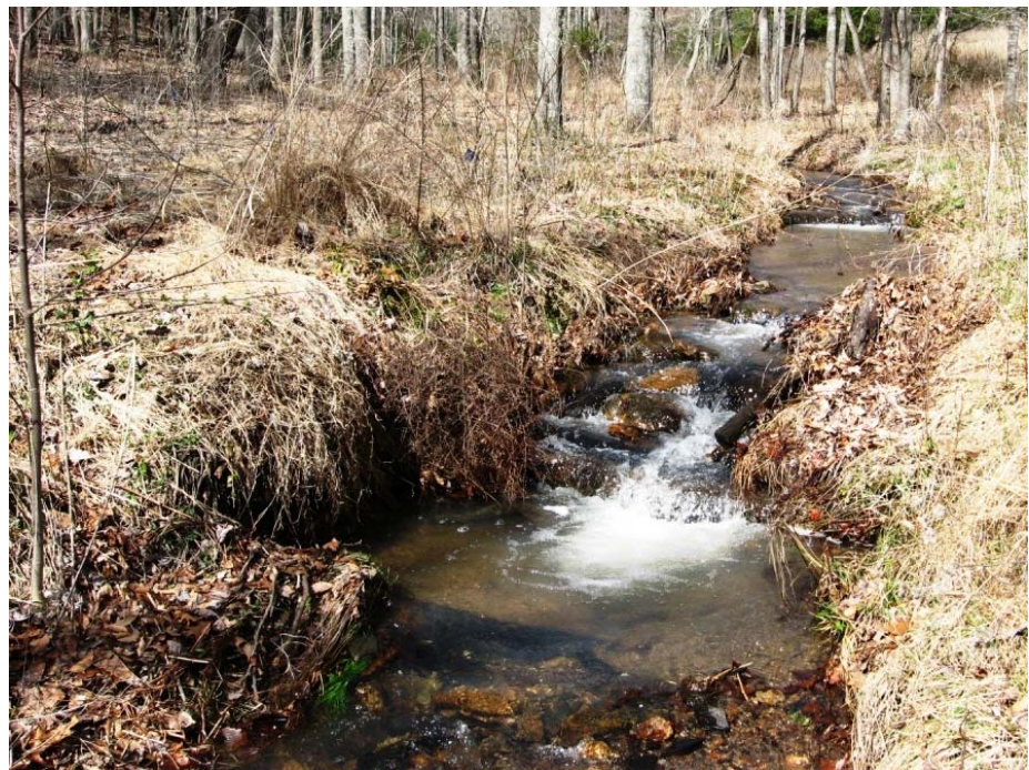
Photo at right: March 7, 2011. This is a view of the unnamed tributary to Purlear Creek, restored during Phase-1 and 2. Note the abundant leaf litter deposited along both stream banks, indicating high water events. Structures remain intact and functioning. Some of the pools are partially filled, as legacy sediment is mobilized downstream through the restored system.
