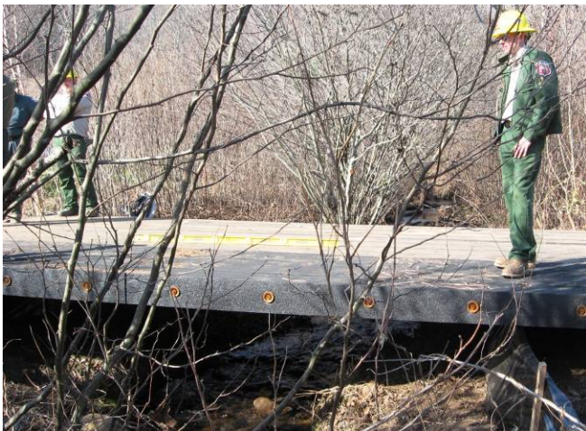
A side view of the installed bridgemat crossing, looking upstream.
