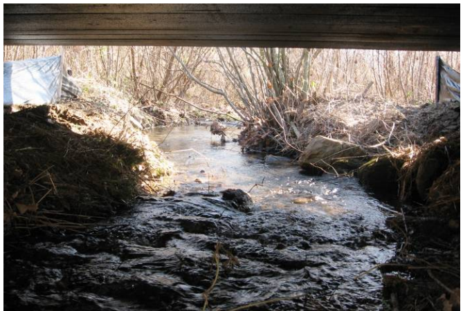
View from underneath the crossing, looking downstream.
