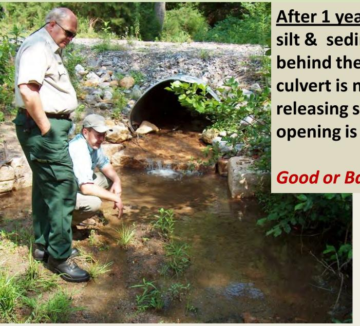
After 1 year: Decades of silt & sediment build-up behind the under-sized culvert is now naturally releasing since the opening is larger.
