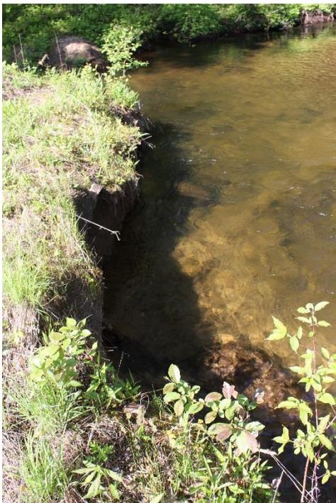
A short segment of the left-bank (estimated 10 feet, see photo at left from May 2015) was observed as washing out, at the point where the restored stream reach ties-in to the legacy (un-restored) channel. We will observe this area and if needed consider actions for curtailing or minimizing continued bank erosion.
