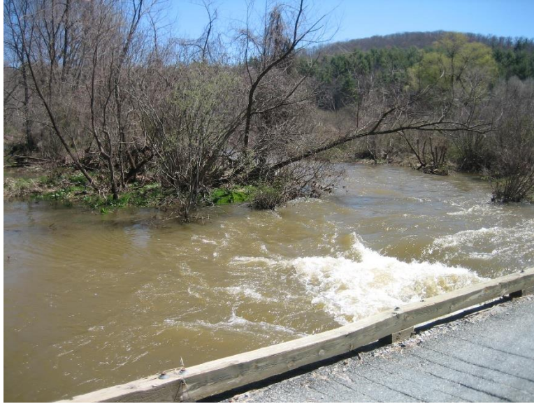
Photo 6: Reach 3, upstream view of mid-channel bar from Greene Road bridge
