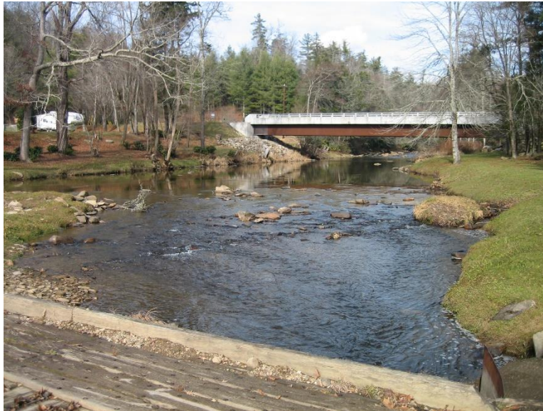
Photo 3: Reach 2, upstream view from low-water bridge
