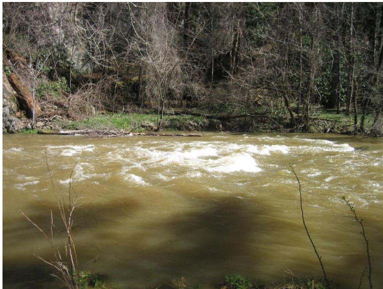
Photo 2: Reach 1, right bank erosion
