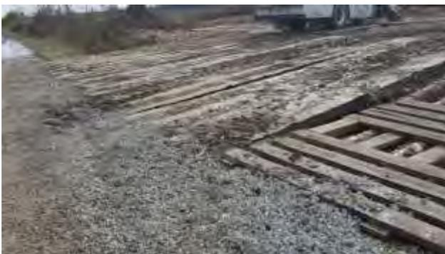
Figure 2: Two perspectives of several bridgemats spanning a road-side ditch in the Coastal Plain of North Carolina
