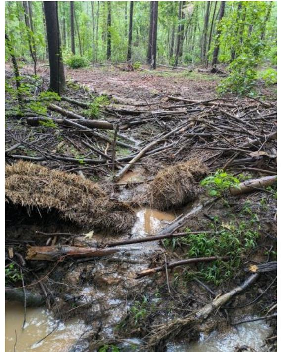
*A closed skid trail shortly after a rain event where straw bales were used to help reduce sedimentation at two different stream crossings.*
