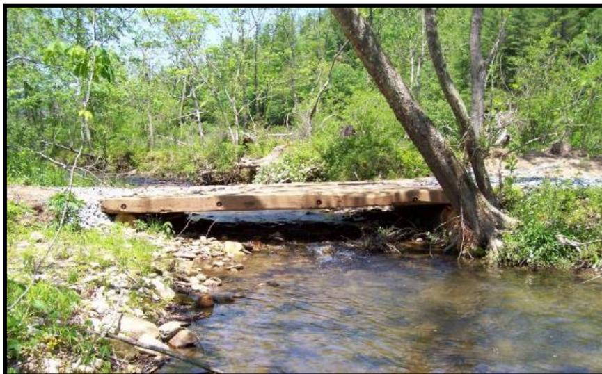
When crossing a necessary stream during forestry operations, a temporary bridgemat, such as the one pictured above, may be used to maximize water quality protection.
