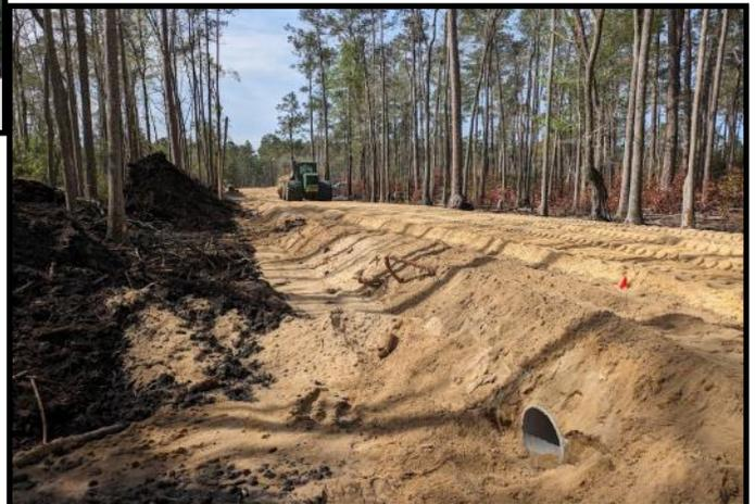
Planning ahead and collaborating with stakeholders has been key to a successful project minimizing the wetland impact and length of a wetland road. The photo above shows the proposed road map identifying BLSF boundaries, soil series and roads. Geotextiles will be used to create a firm road bed in mucky soil. The photo to the right is first construction of the wetland road in March, 2024.
