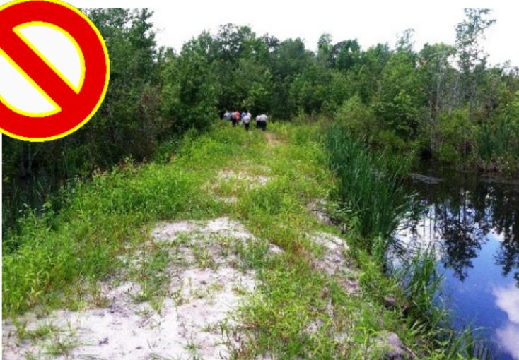
This is not an acceptable wetland forest road. Water is backing up (on right) and the road is not wide enough to support logging trucks. There is not enough groundcover stabilization to minimize soil erosion.
