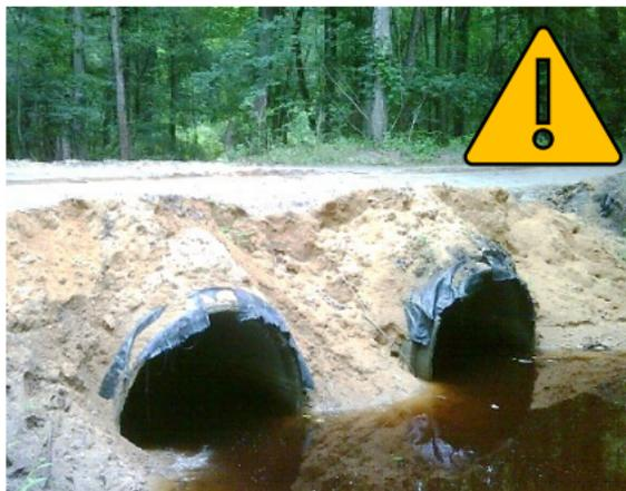
This culvert crossing in a swamp needs stabilization of the newly applied backfill.
