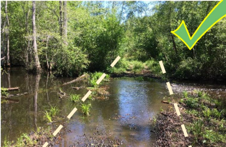
This rock ford on a wetland road allows water to pass.
