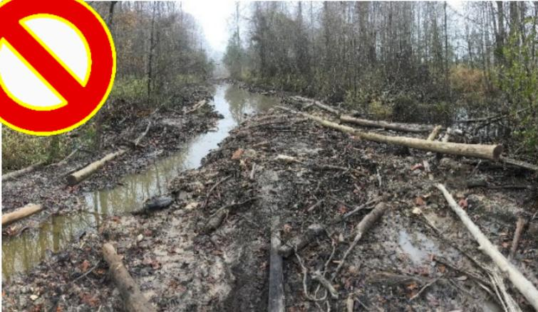
This wetland road is in unacceptable condition after logging. Debris must be removed. The road needs reshaping to allow water to pass and groundcover to stabilize the soil.
