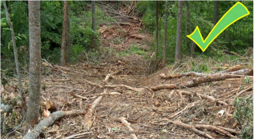
This overland skid trail uses slash to control the runoff and erosion on the approach way to the stream crossing.
