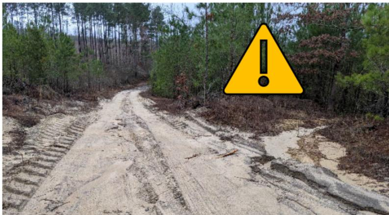
Low standard roads like this often need more work to maintain surface drainage and erosion control structures.
