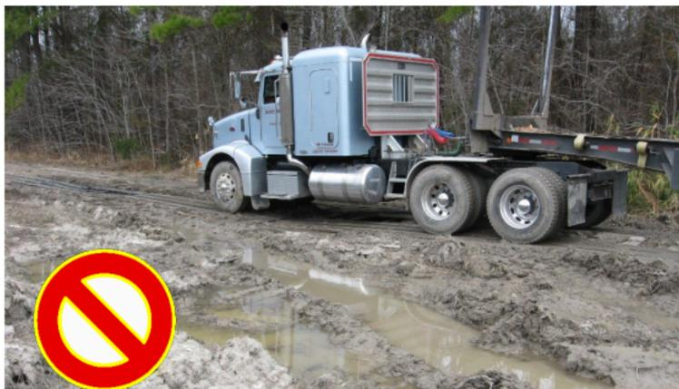
This road is sloppy and has lost its structural integrity. Sedimentation into streams is very likely and extra wear and tear on equipment is possible.
