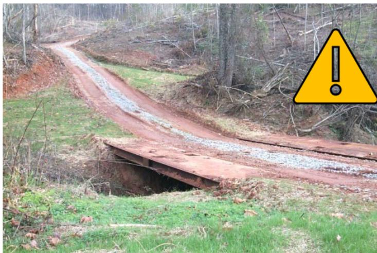
Good road using gravel, diversions, grass and bridgemats. Work is needed to level off the ruts and prevent sedimentation runoff into the stream.
