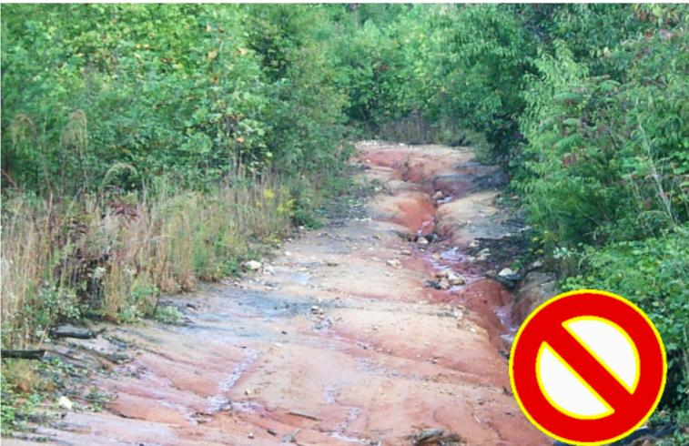
An erosion gully is carving away the road because it lacks water diversions and surface stabilization.
