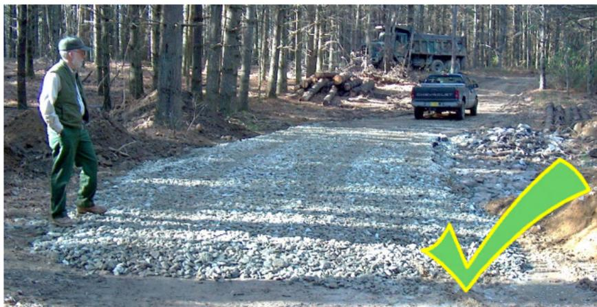
An ample layer of stone promotes surface drainage, good control of runoff and improved trafficability.
