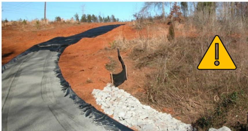
Geotextile keeps gravel from sinking into soft soil. Curving the road reduces the grade and gives room to install water diversions. Groundcover is needed on bare soil.
