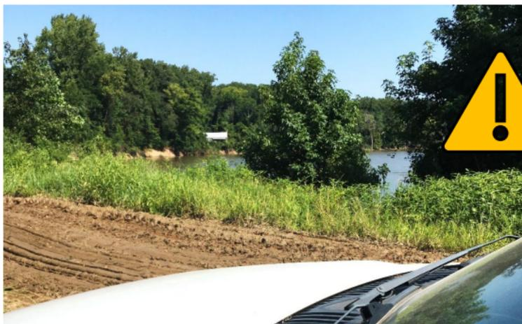
This road is too close to a large river. The narrow strip of weeds is the only thing keeping sediment out of the water.
