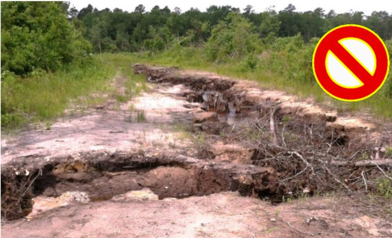
This road was blown out because of inadequate cross drainage to handle storm runoff from neighboring land.
