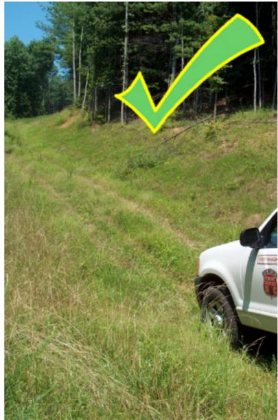
**LEFT:** No diversions or groundcover, resulting in accelerated erosion and gulying of the road.
