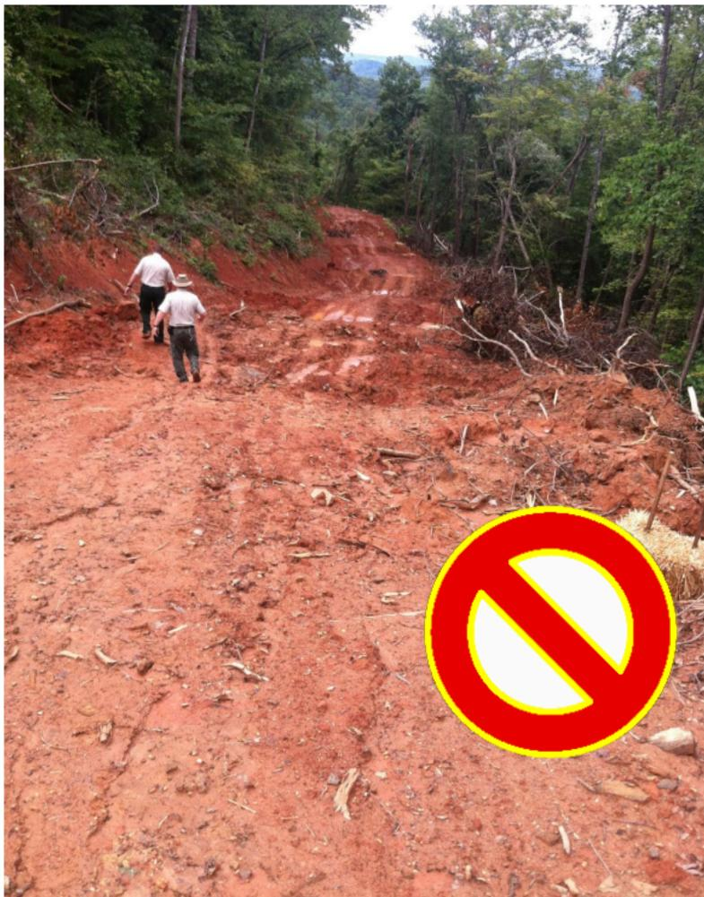
Little effort went into installing water diversions. Too much soil was exposed all at once with no groundcover. Construction was during a wet period and it was used too soon, with no time for it to firm up.
