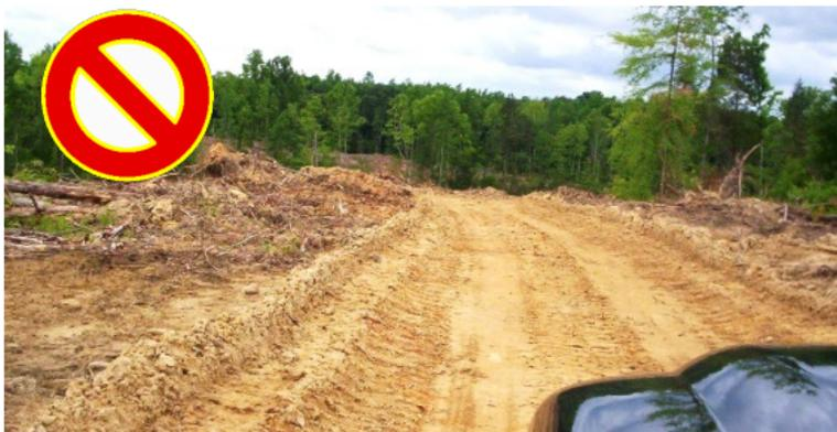
Soft soil has been repeatedly scraped off this road, creating side berms of soil that trap rainfall runoff. Significant regrading is needed to reshape this road.
