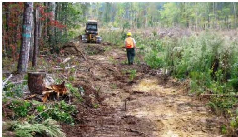
A skillfully bladed fire line for a site prep burn.
