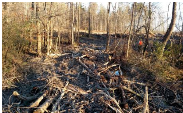
Stream crossing approaches stabilized with brush. Photo courtesy of N.C. Forest Service.
