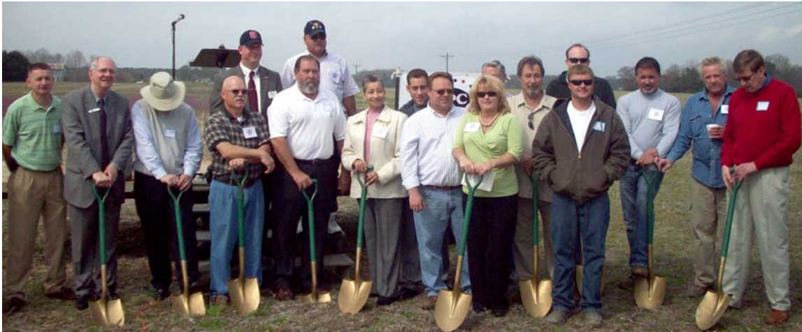
APC members and supporters from county and state agencies at the ground breaking for APC's new processing facility. Photo courtesy of Charlene Jacobs
